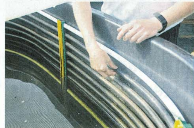
Heating elements inside a fish tank, more effective than simply using the air in the greenhouse.
